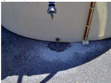
problems caused by exceeded numeric action levels (NALs). A little tightening of this tank bung and cleanup of the surrounding pavement could save literally hours of your own time and thousands of dollars responding to exceeded NALs. Prepare for this year's coming rain by carefully inspecting your industrial facility and making a note of any items similar to this one that need repair or maintenance. Coordinate maintenance and cleanup efforts to occur before the first rain of the season.
