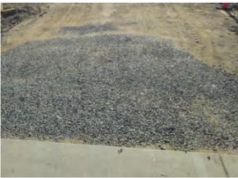
longer be effective such as the track out control shown here. Track out controls lose effectiveness every time a vehicle passes over it or a gust of wind blows sediment onto it. Some BMPs are seasonal. This track out control might
