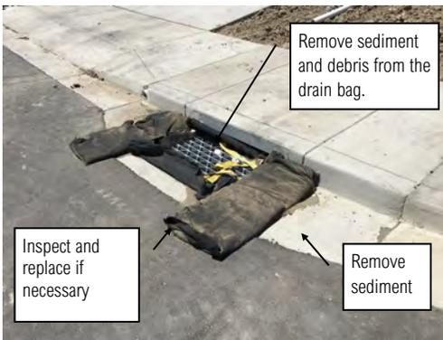
Drain inlets need to be inspected for a build up of sediment accumulated from wind and dry season construction activities. If a geotextile or plastic barrier was installed under the grate, remove it and replace it with a drain inlet bag insert. Refresh gravel bags (or compost socks)
