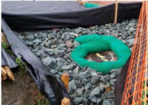
extremely important (it can be square or triangular), it is a good idea to include geotextile fabric inside the silt fenced area and cover it with some rock. (This particular photo also includes a compost sock or Type 7.) However, please remember that silt fence is not very permeable and you could get some flooding outside it. **TIP:** to alleviate this,
