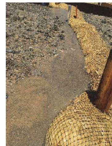
2. We observed that wattle used as a linear break can handle a significant amount of precipitation.
