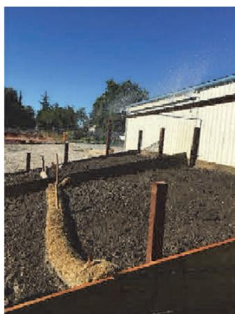
But, does wattle work when it is properly installed? To answer this question we set up a demonstration in our **Construction Sandbox**. We installed a section of wattle on a 25% slope. The installation was per CASQA / [Caltrans specs](#), keyed in 2 – 3 inches deep, and staked. We then subjected the wattle to heavy “storm events” of 2” and more than 6” and watched
