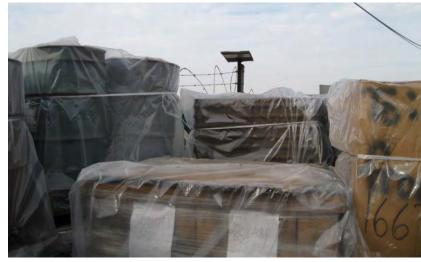
cover seen here can be created using plastic sheeting which is readily available from your local hardware store. One challenge is keeping the sheeting securely in place especially during windy conditions. An innovative product, called the Symmloc fastener, can be
