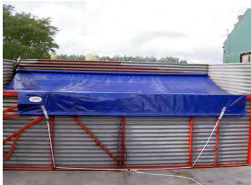
Using what you have learned from the evaluation in step 1, begin to develop mitigation measures to improve on areas that were identified. Where feasible, move pollutant generating activities and sources under cover. Cover can be as complex as building a structure to provide area coverage or as simple as securing a tarp over sources (i.e., metal recycling bins).
